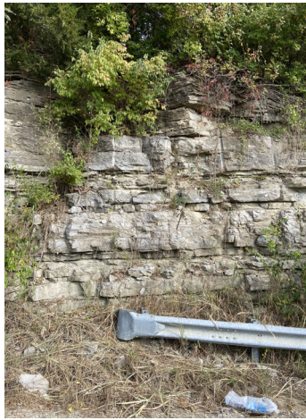
Figure 2. Lexington Limestone on KY 52 west of Dix River crossing
