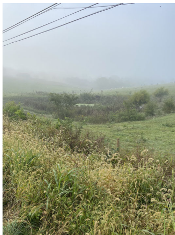
Figure 3. Water filled sinkhole south side of KY 52 in Boyle Co.
