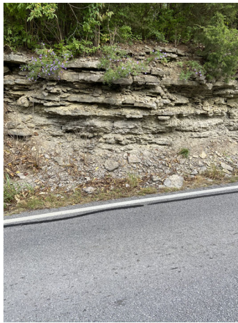
Figure 5. Rock cut east of the Dix River
