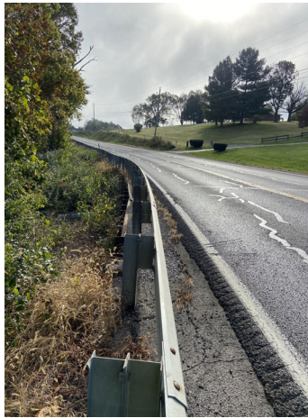
Figure 6. Rails and lagging mitigation on embankment east of the Dix River
